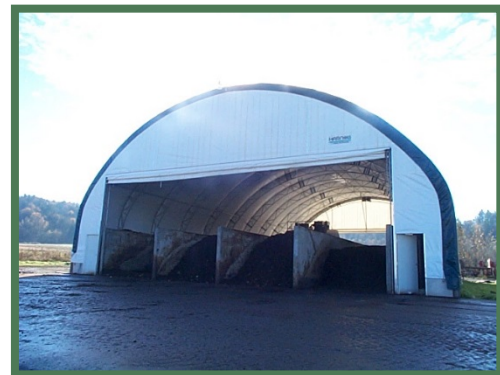
Figure 7: Channel Compost System
