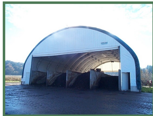
Figure 7: Channel Compost System
