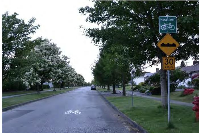
The desired road clear width for shared lane bicycle routes is 5.5 m, and a minimum of 4.3 m in constrained circumstances. Traffic characteristics of shared lane bicycle routes are an essential consideration and will only be accommodated on roads with fewer than 500 vehicles per day, desirably fewer than 500 vehicles per day. Since they are most likely to be located on local roads, shared lane bicycle lane routes will be accommodated on asphalt surfaces.
