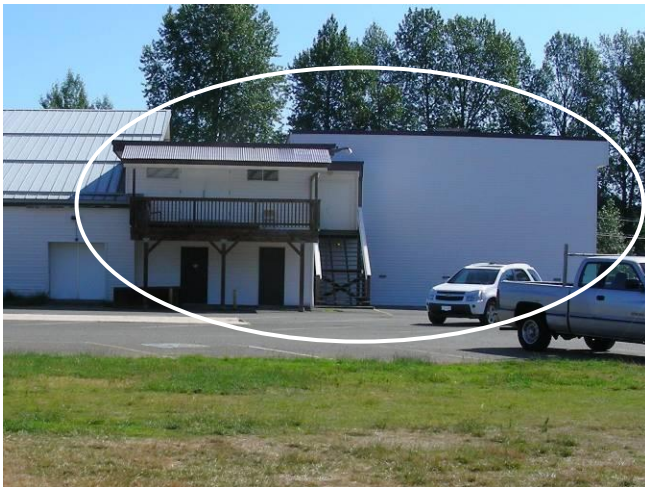
Fig. 1.4.6 View of the Social Component of the Facility.
