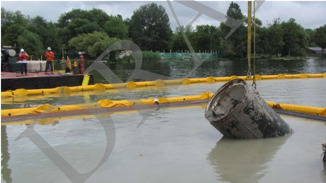
Figure 5-5: Removal of MTBM Within Turbidity Curtain
