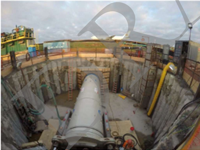
Figure 5-3: MTBM Launched Under the Runway at Pearson Airport
