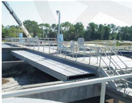
SureGrip beam-supported splash cover Racetrack Aeration Basin
