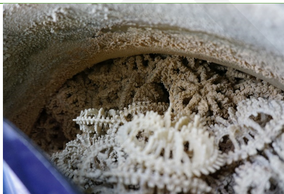
Existing Scrubber Media: Jaeger Tripack with solid deposits at central section of the scrubber vessel.
