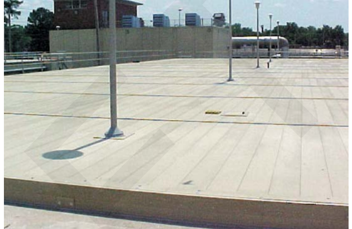
SureGrip beam-supported tank cover system Sedimentation Basin
