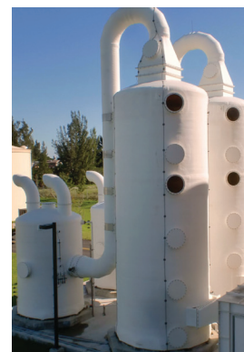
Carbon Adsorbers used as polishing units following a Biotrickling filter.
