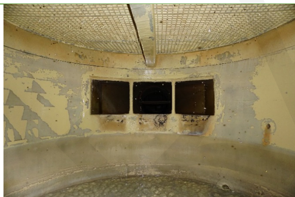
Internal wall of the existing FRP scrubber vessel (below scrubber media section).
