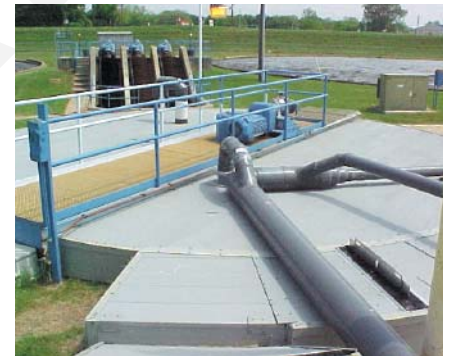
SureGrip beam-supported cover - 31' diameter Grit Basin
